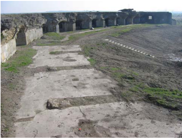
5 April 2008, with the earth ramp in place
