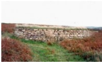
Wall surrounding dangerous mine shaft, North Cornwall Coast
