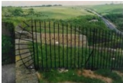
Railings at Dover Castle
